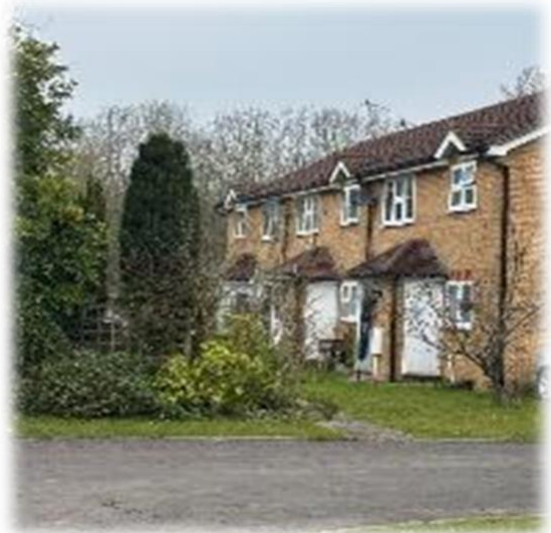
Alberta Drive Terrace
